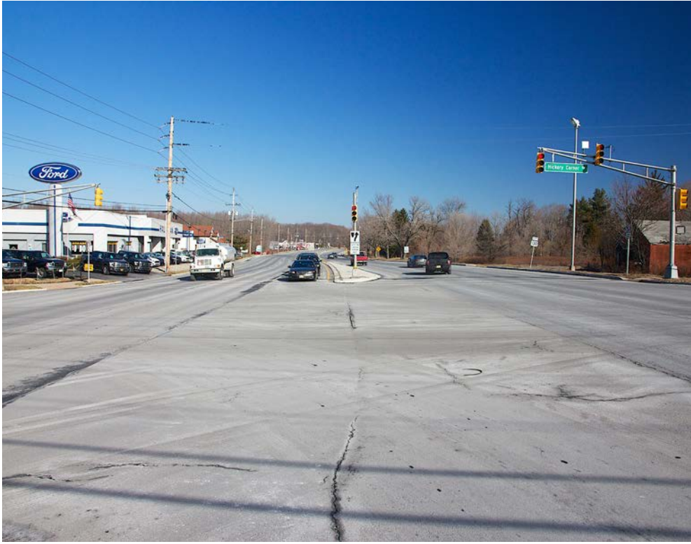
U.S. Route 130, facing north
