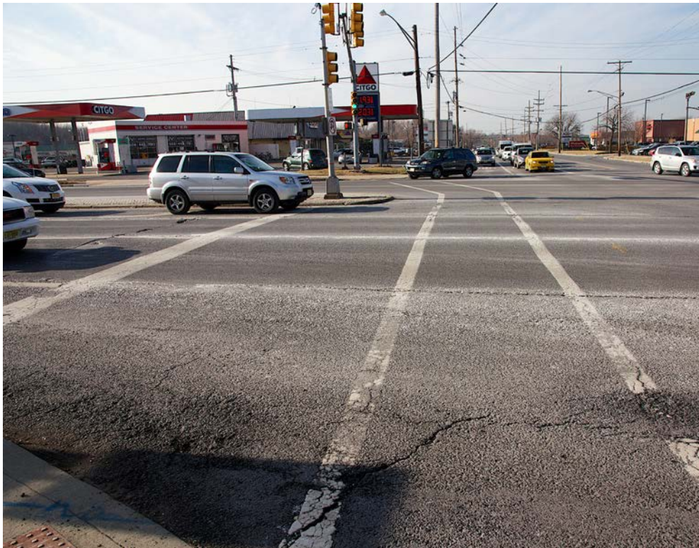
SE corner, facing west
