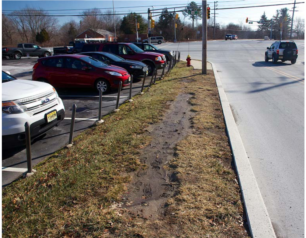
Worn path and utility obstruction along Hickory Corner Road near U.S. Route 130, facing east
