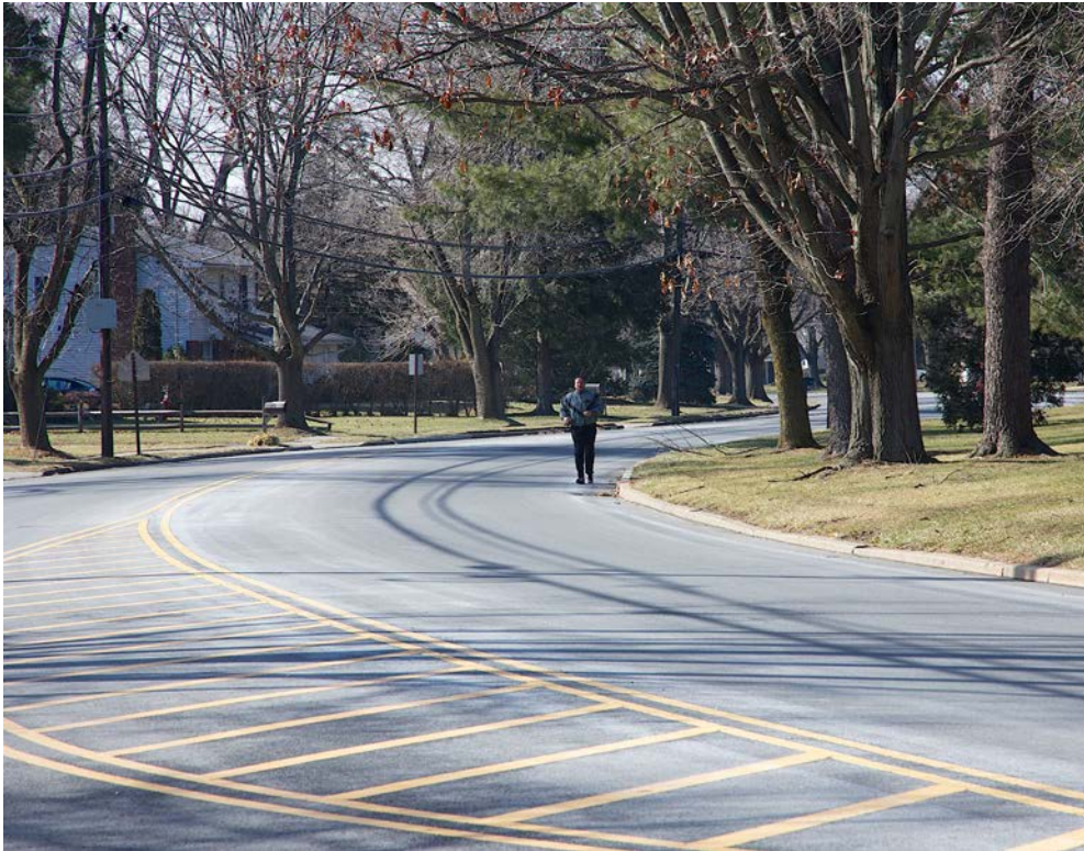
Dutch Neck Road at Oak Creek Road, looking west
