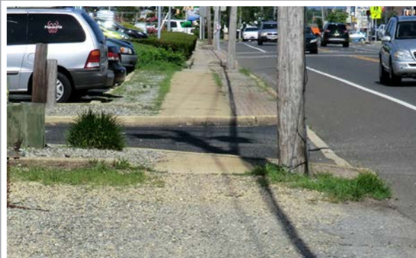
Wrong: Driveway cutting through sidewalk
