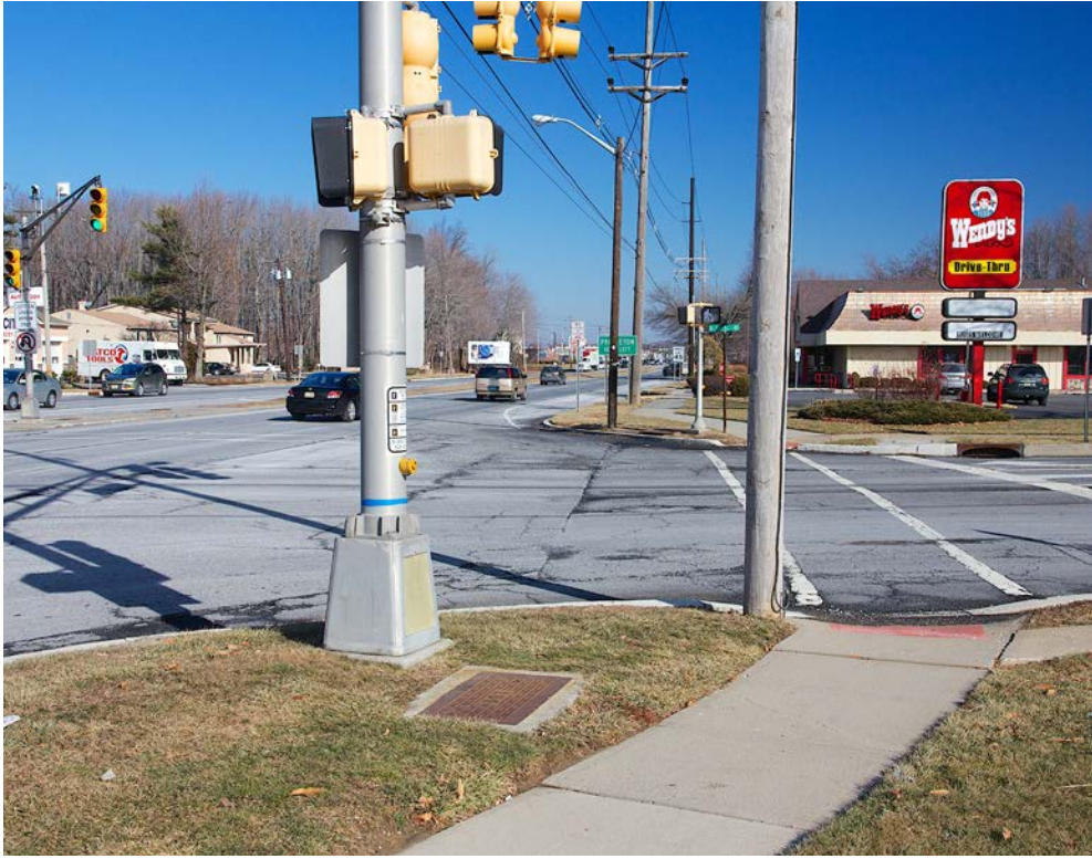
Pedestrian push button not accessible from crosswalk on SE corner, facing north
