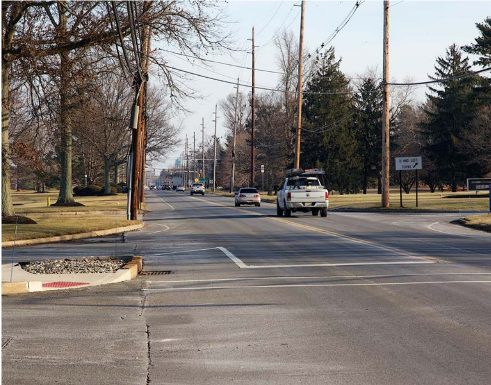
Princeton-Hightstown Road at McGraw Hill, looking southeast
