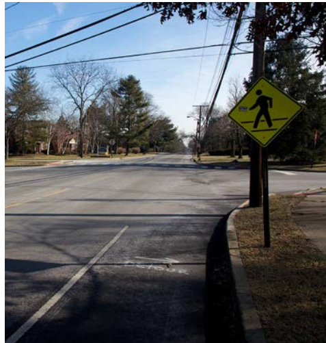
Left: Missing sidewalk connection along Hickory Corner Road, facing west
