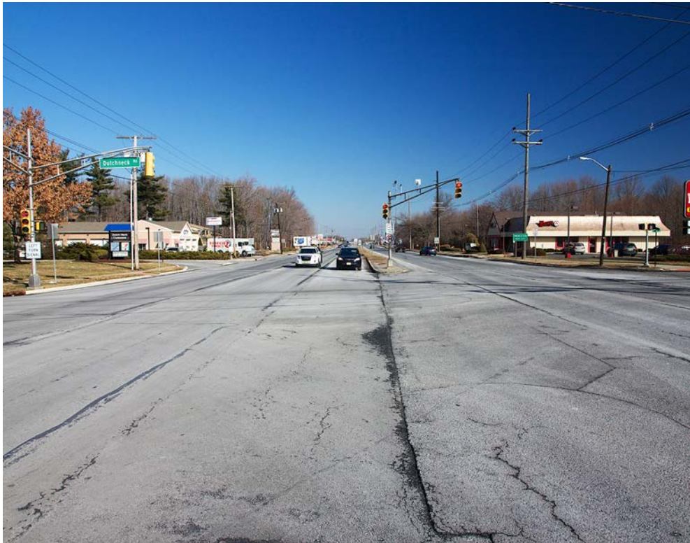
U.S. Route 130, facing north
