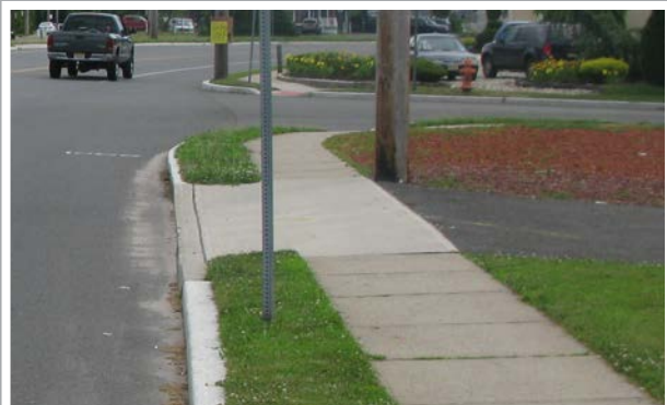
Right: Sidewalk built through driveway
